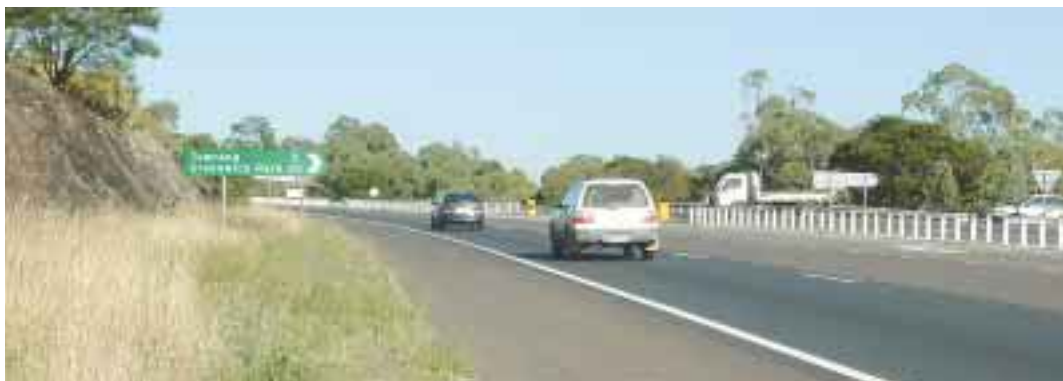
The dangerous intersection of Towrang Road and the Hume Highway will receive a $5 million upgrade.
